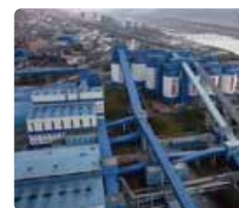
Daliuta Coal Mine Industrial Park Yulin, Shaanxi
