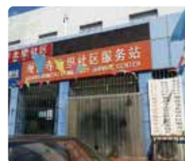
Smart Fire Protection Renovation Project of Guanyinsi Community, Daxing District, Beijing
