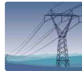
Smart Fire Protection Renovation Project of State Grid Jibei Electric Power
