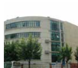
Smart Campus Project of Jing'an District Education Commission Shanghai
